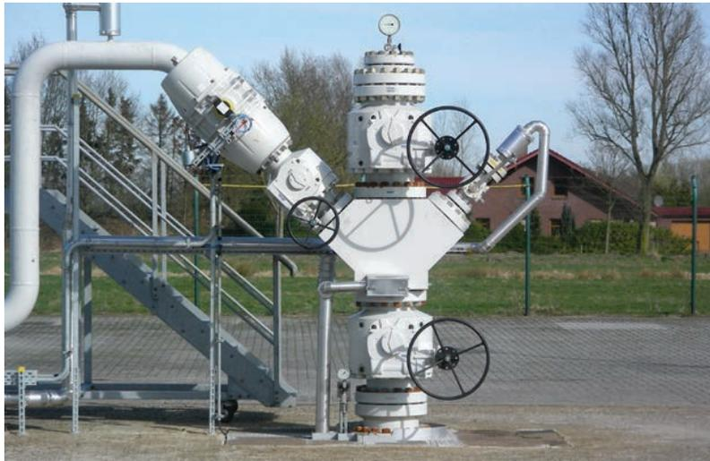
Reliable combination: Hartmann gas wellhead with gas-tight, metallic sealing ball valves in Jemgum, Germany.
